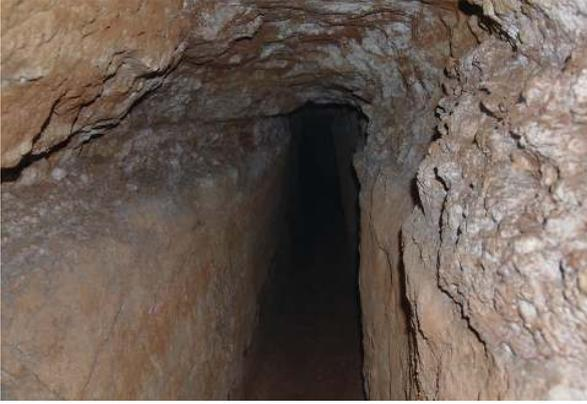
Fig. 12 The *adit* at Bureta is some 100 m long, 2 m high and 0.9 m wide.
