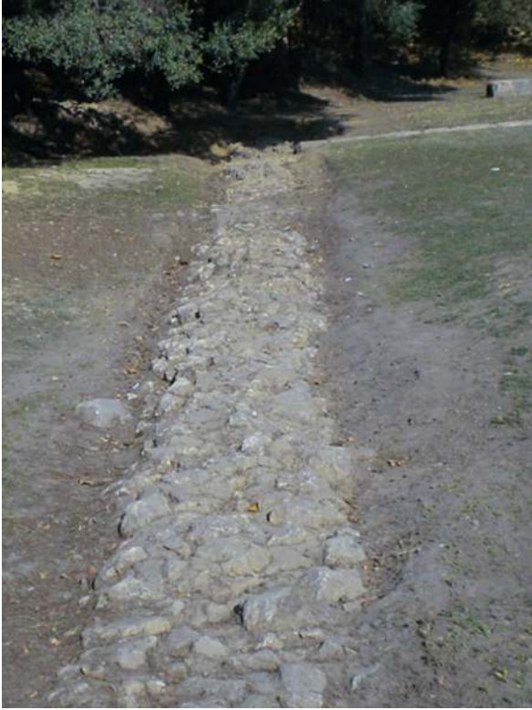
Fig. 6 Athens, Academy, so-called gymnasium: foundations on the east side of the courtyard, detail of the building material.
